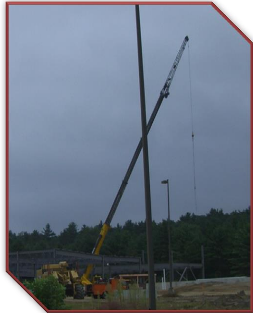
Figure 7: Telescoping Crawler Crane used on site
